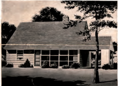
REAR VIEW OF ALL HOUSES
